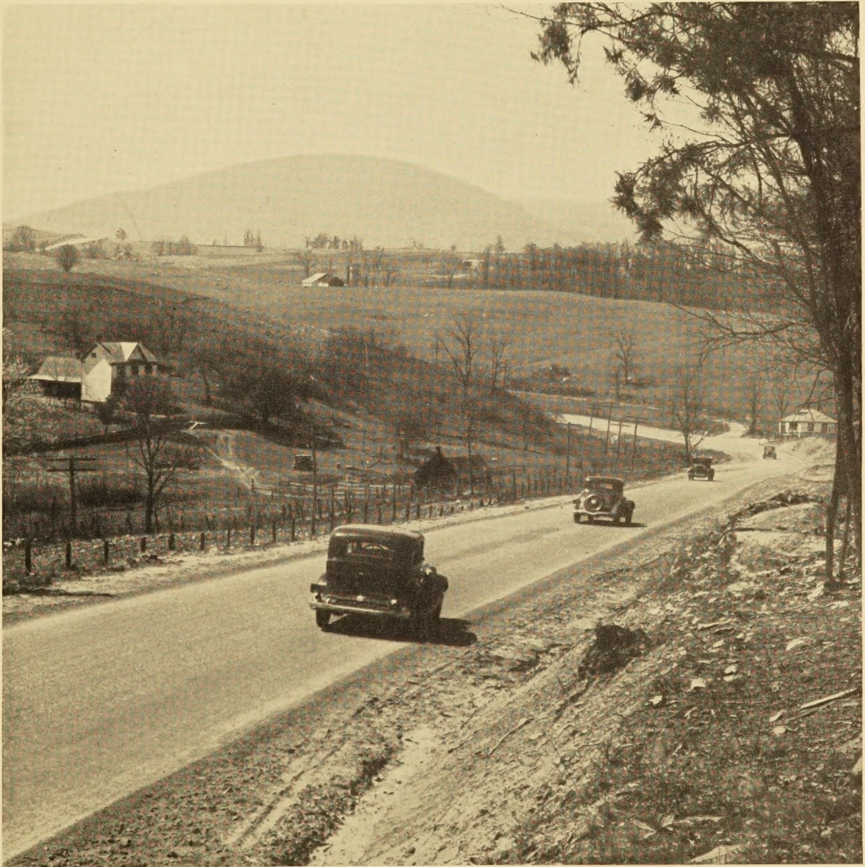
A STABILIZED SOIL ROAD IN VIRGINIA
